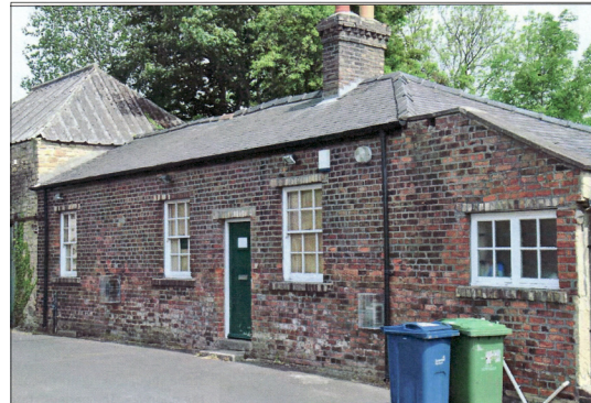
This rubble stone building probably dates back to the very early 19th century. It has a hipped roof (4 surfaces) covered with 20th century asbestos. It was probably originally used to house a horse(s) and a carriage with a hay loft above.
