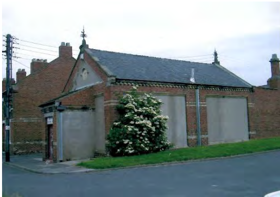
Hetton Band Hall prior to demolition.
