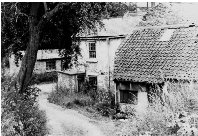
Bleach Green first a brewery then a smithy, but now demolished.
